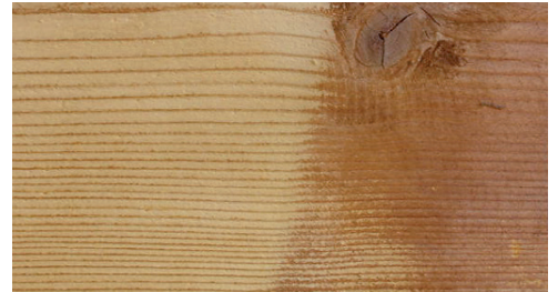
Wooden façade before and after cleaning
